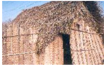
A new thatched roof hut
